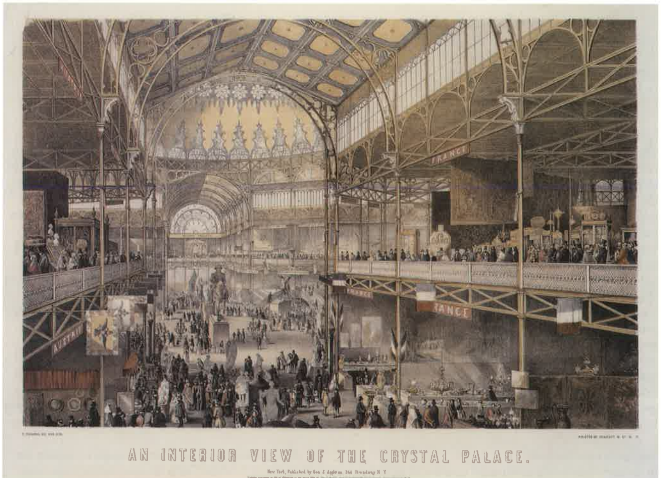
Fig. 3: Interior of the Crystal Palace in 1853, the year that the building was completed. It hosted the American Institute exhibitions from 1853 until it was destroyed in an 1858 fire. Courtesy of the New York Historical Society. Negative no. 167.
